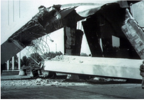
Congress Hall in Berlin after the collapse.
